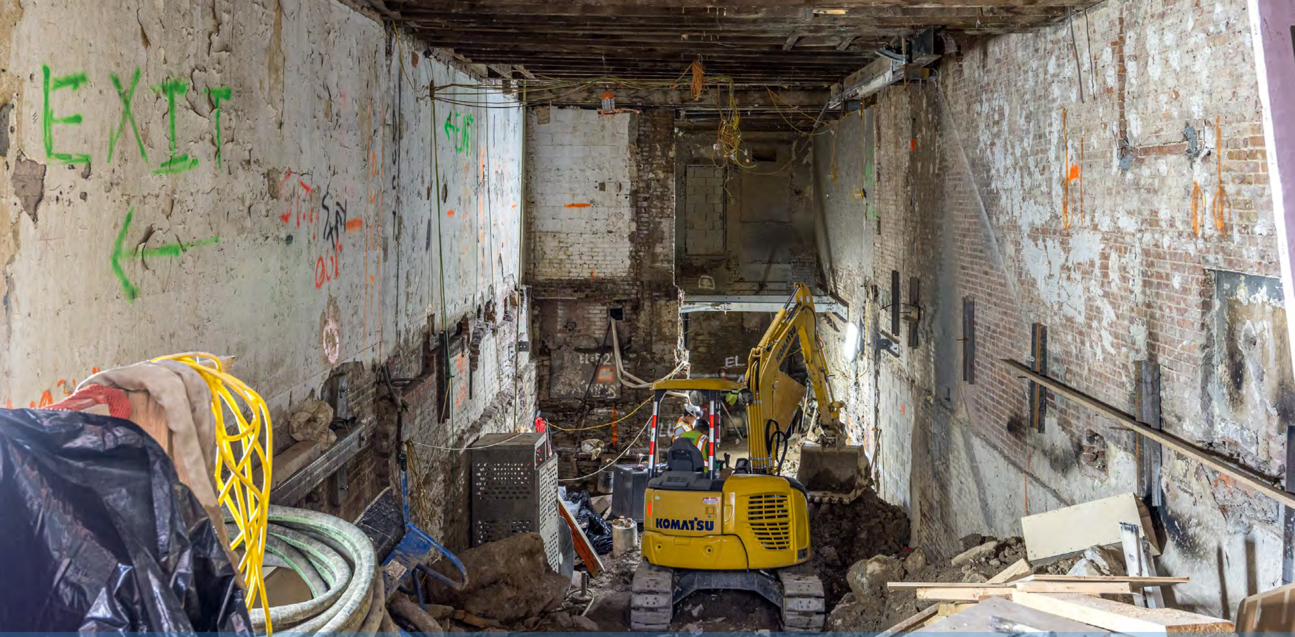
EXCAVATION UNDERWAY AT 762 MADISON
