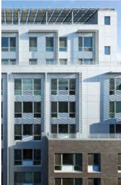
Rooftop solar canopies
