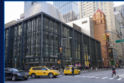
FULTON TRANSIT CENTER
