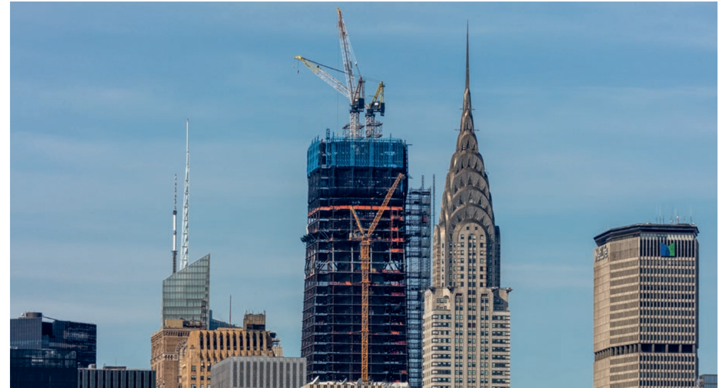
One Vanderbilt construction progress
