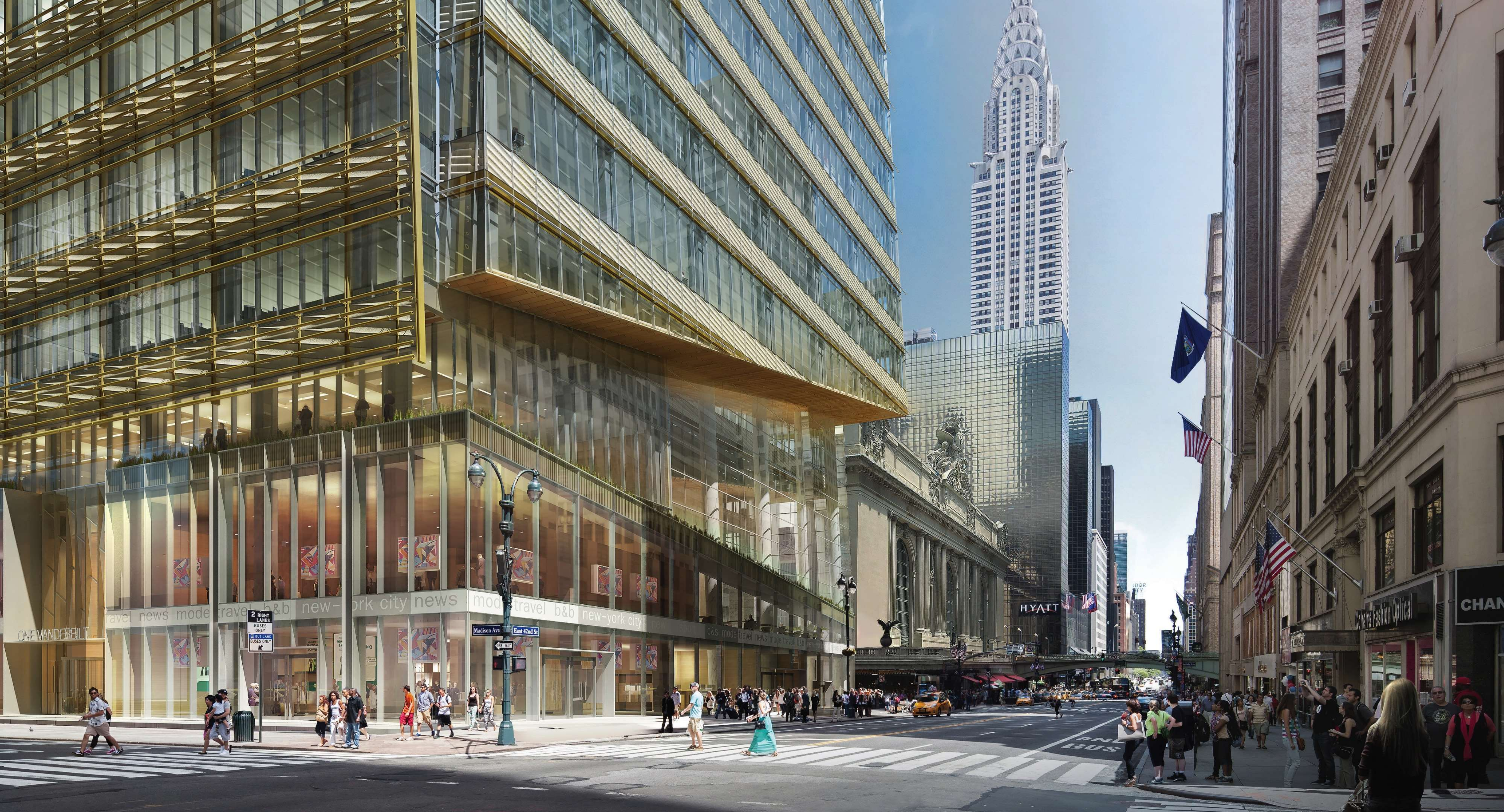
LOOKING EAST FROM 42ND STREET
