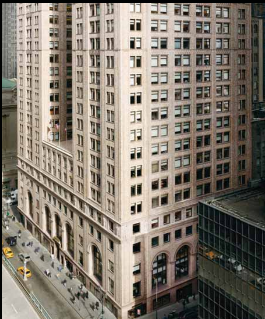
Top: One Madison Avenue. The centerpiece of Midtown South and part of Credit Suisse Securities (USA) Inc. headquarters campus.
