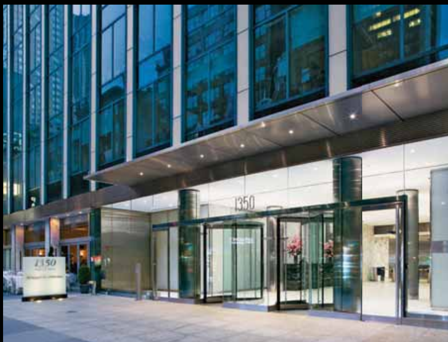
Top: One Hundred Park Avenue. Recipient of BOMA's 2009 International Building of the Year Award for its renovation.
