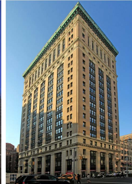
315 Park Ave. South
